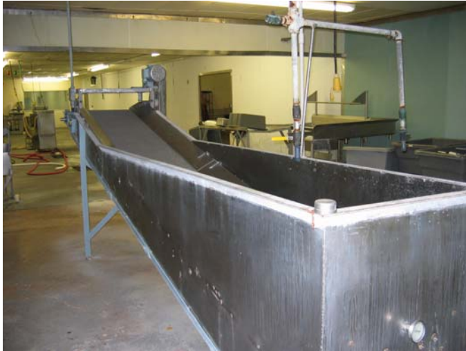
7. All Stainless Steel Holding Tank
